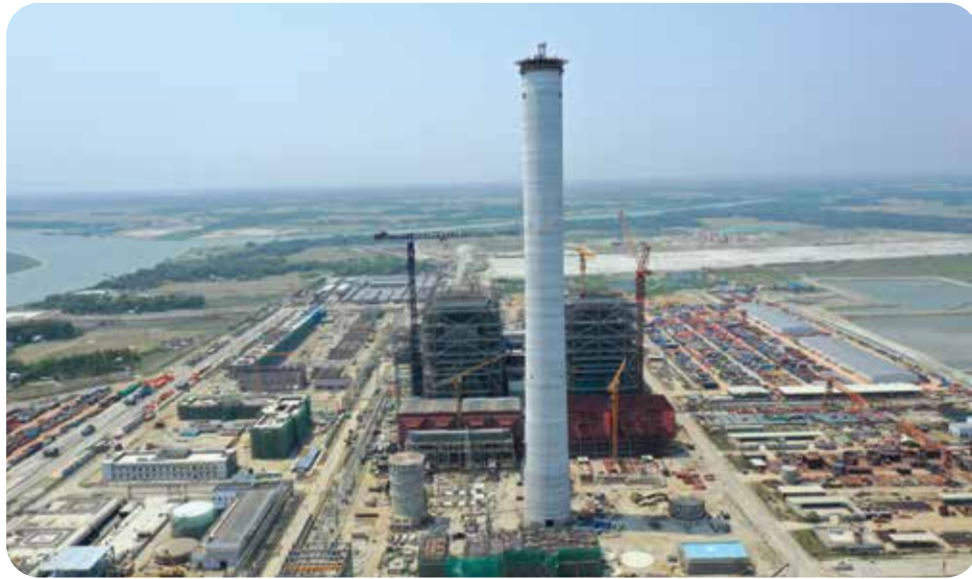
Chimney : Payra 1320 MW TPP Project (1st Phase)
