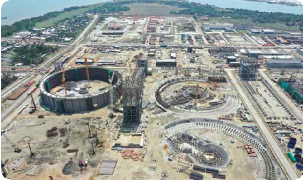
Coal Yard : Payra 1320 MW TPP Project
