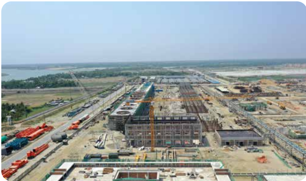
IDCT : Payra 1320 MW TPP Project (1st Phase)
