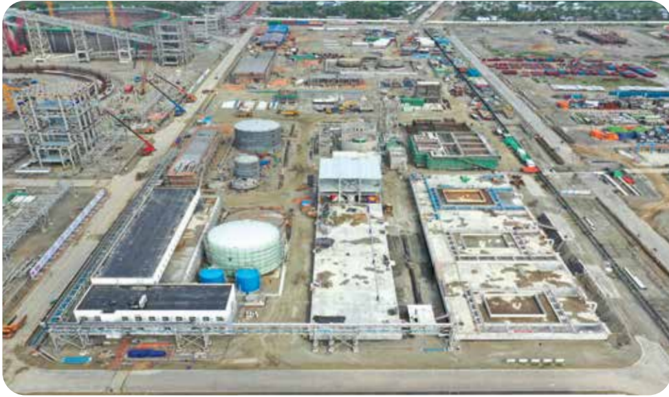
BOP : Payra 1320 MW TPP Project (1st Phase)
