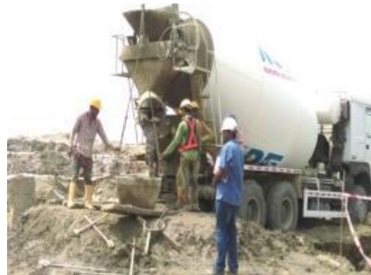
NDE Workers with PPE
