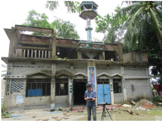
Noise Level Monitoring at Char Nishanbari Mosque
