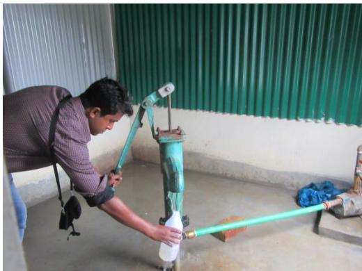
Ground Water collection at Project Area
