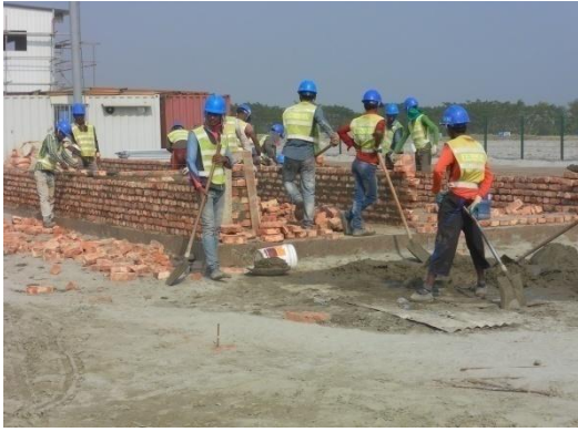
Working with PPE
