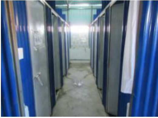
NEPC laborers toilets facility
